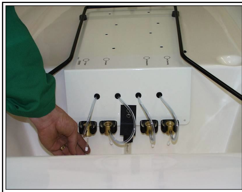
Figure 4.3.1 Preliminary Installation of Aroma System.
