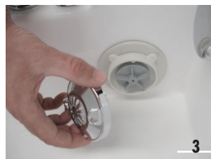
Pict.7 Cleaning of the whirlpool tub impeller
