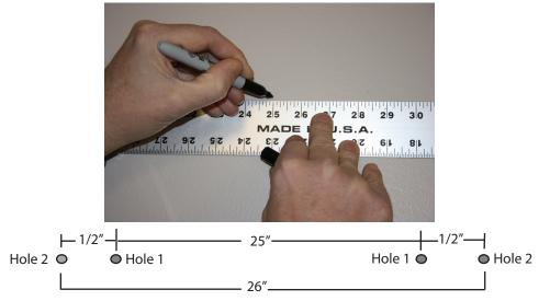
If the surface is hollow, drill 3/16" diameter holes and pound plastic anchors into each hole (see picture below). If surface is solid, drill 3/32" diameter holes.
